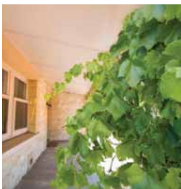
89 ADELAIDE ROAD, MURRAY BRIDGE
